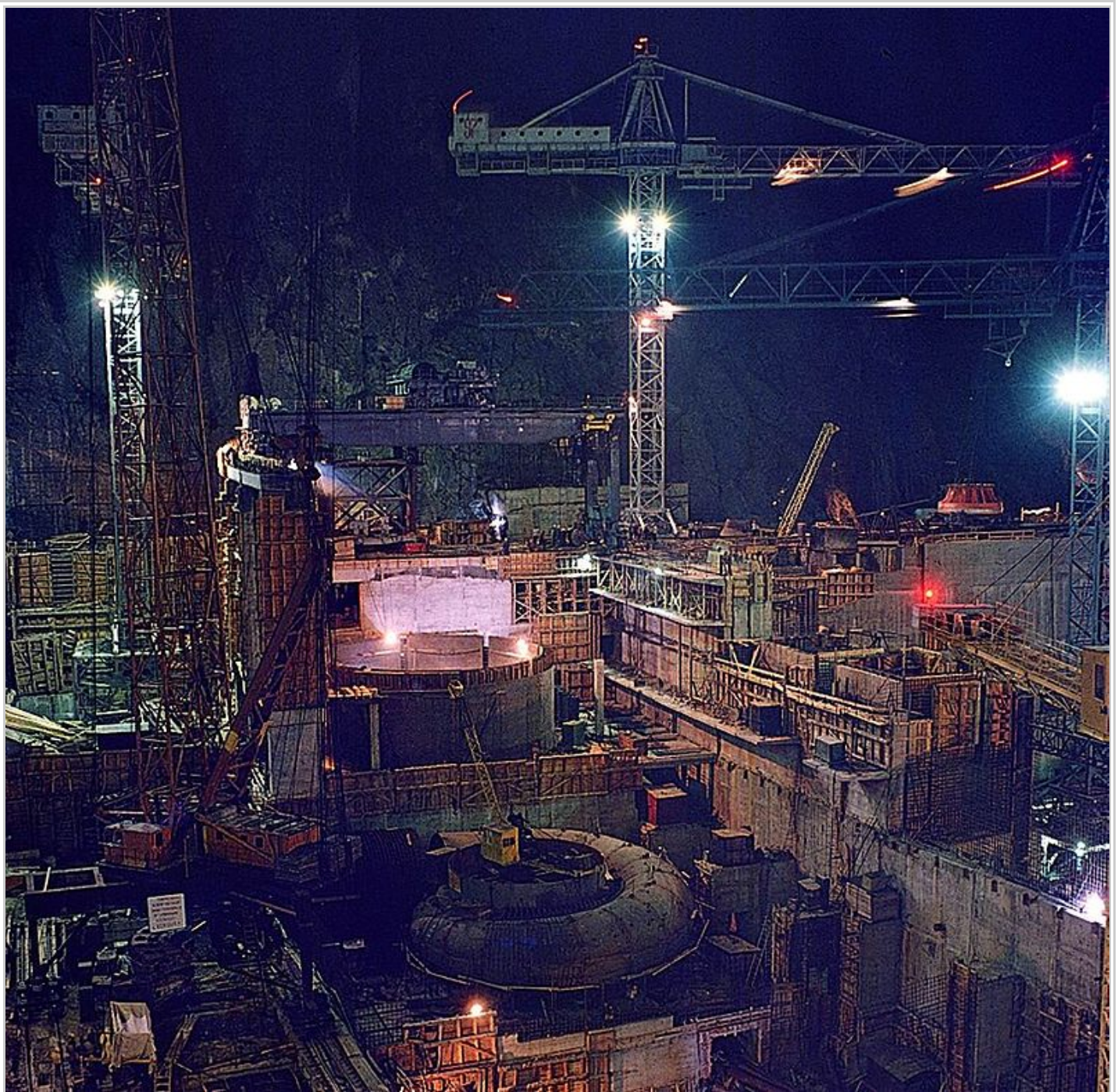
Rice. 3.6 appearance of the camera # under construction of spiral -2 during installation
